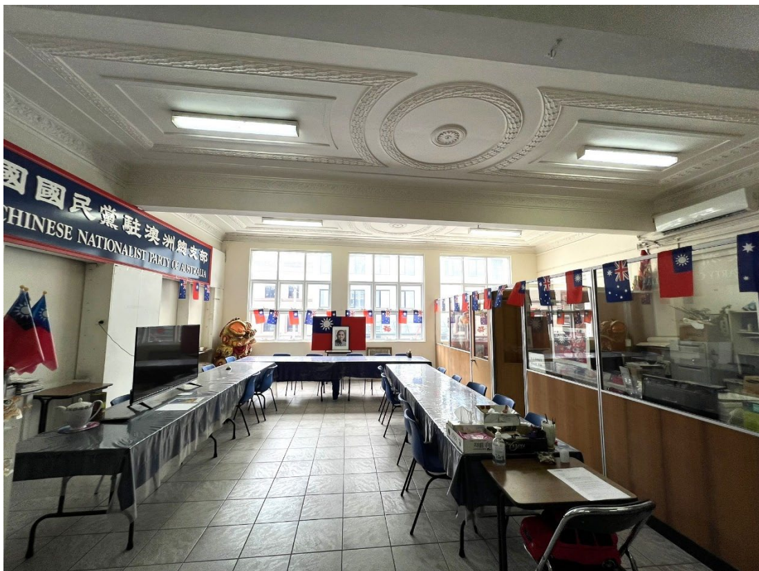
Figure 15 First floor office with plaster ceiling.
